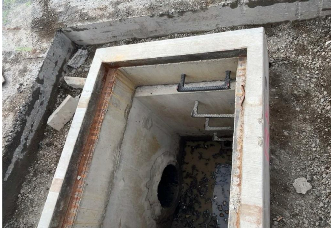
Saw Cutting Existing Pavement to Raise Drainage Inlets
