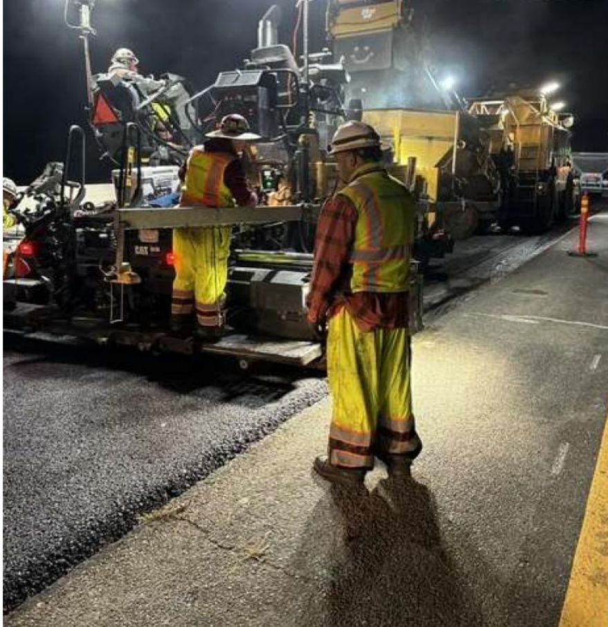
Paving Median Shoulder
