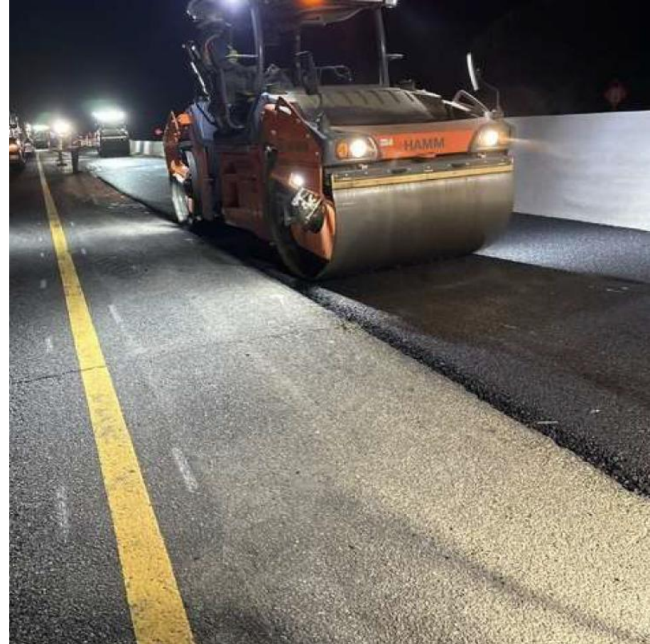
Paving Median Shoulder
