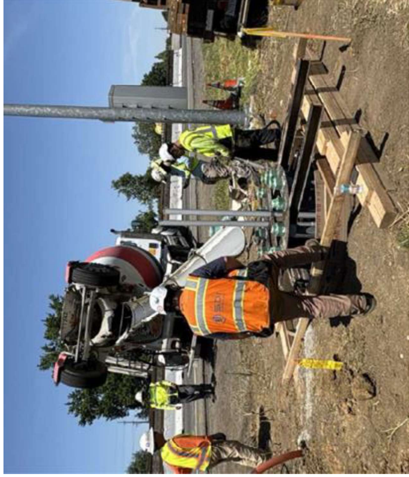
Cast-In-Drilled-Hole Pile Foundation
