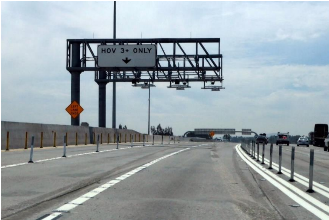
Figure 21: Example - Facility with Channelizers
