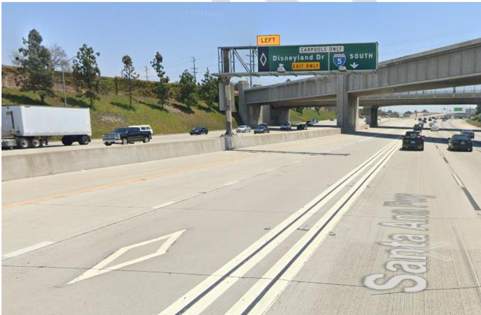
Figure 20: Example - Facility with Painted Buffer
