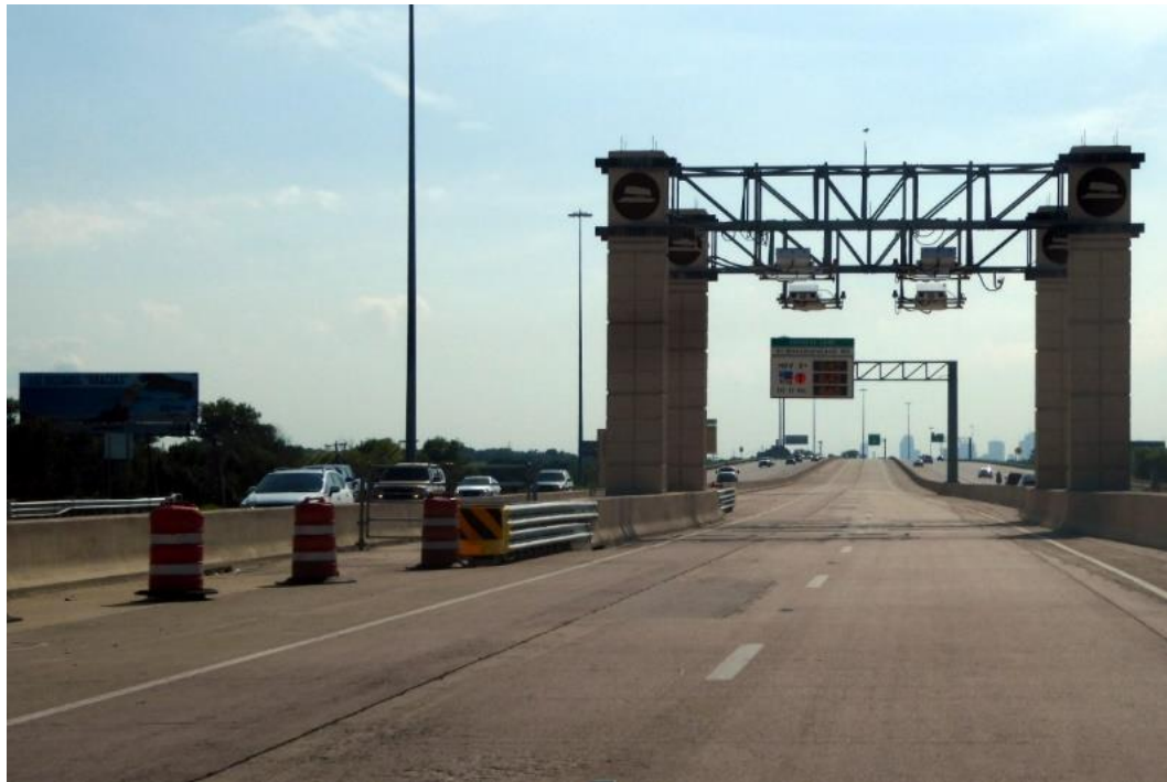
Figure 22: Example - Facility with Concrete Barrier
